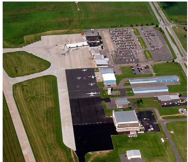
Central Wisconsin Airport
